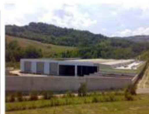
Centralized industrial plants
