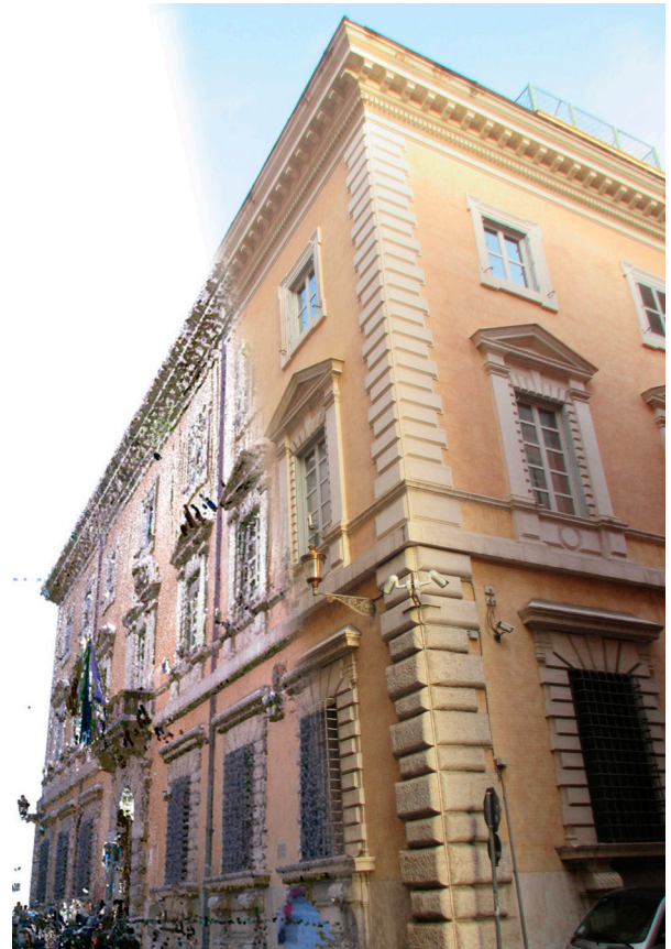
Fig. 1 Palazzo Maffei-Borghese - blending of point cloud and photo.
