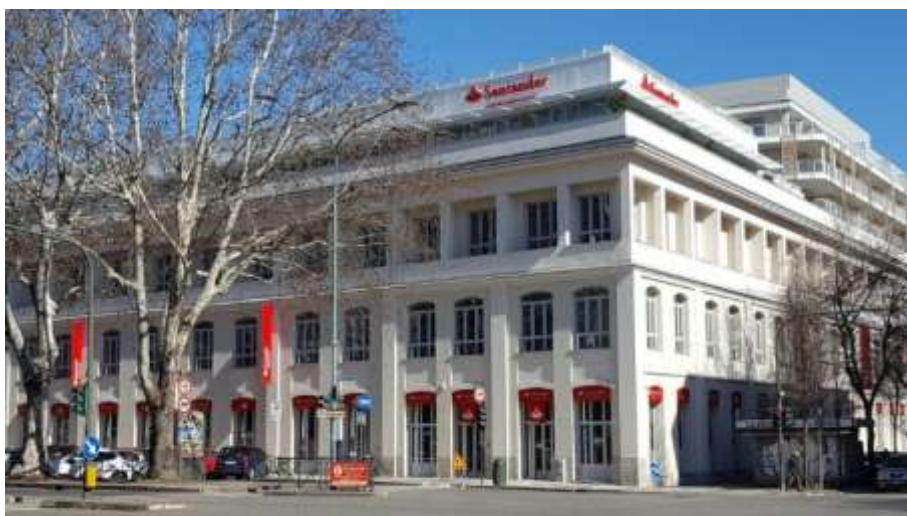
Figure 7: Palazzo Santander. Source: https://citynews-torinotoday.stgy.ovh/~media/original-hi/9040049169856/palazzo-santander-2.jpg
