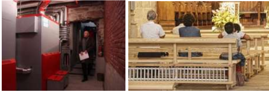
Fig.09: Biomass heating system at the Real Colegiata de San Isidoro (León). Sources: https://www.diariodeleon.es/articulo/cultura/san-isidoro-estreno-pionero-sistema-calefactor-biomasa/200912180332001072894.html - https://decoracion.tendencias.com/varios/la-novedosa-calefaccion-de-san-isidoro-de-leon-eficiencia-y-diseno
