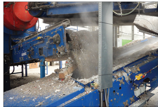
Removal of ferrous material through Magnets
