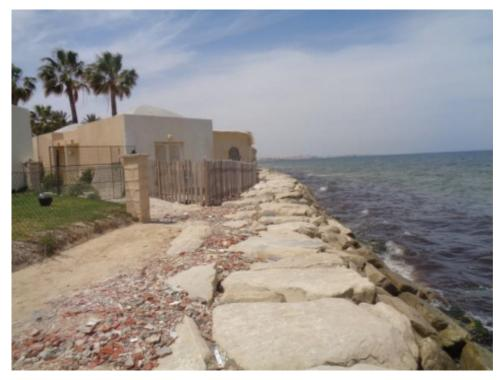
Figure 9. Establishment of a clogging work to protect the arrangements affected by erosion (2015) (Brahim, 2017).
