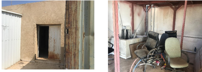
Picture 13: Potential place for solar thermal equipment installation
