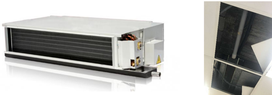
Picture 8: Fan coil units in the roof of the floors
