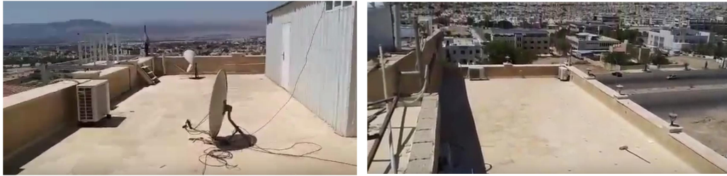
Picture 12: Available place for the solar collector field on the roof of the building (SW and NE sides of the roof)
