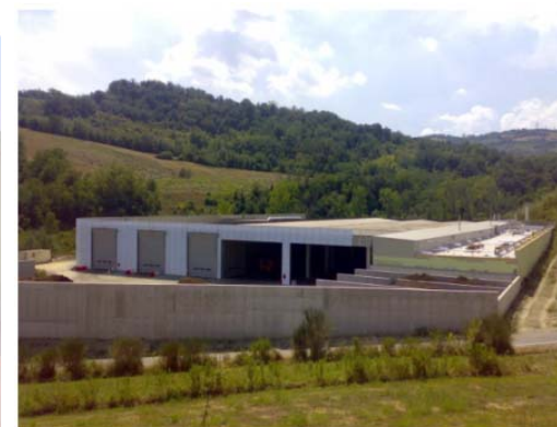
Centralized industrial plants
