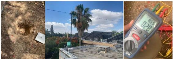
27-Finally the energy meters was installed and configured with monitoring portal – **isolarcloud** for performance monitoring, condition monitoring and data reporting and weather sensor station was installed.
