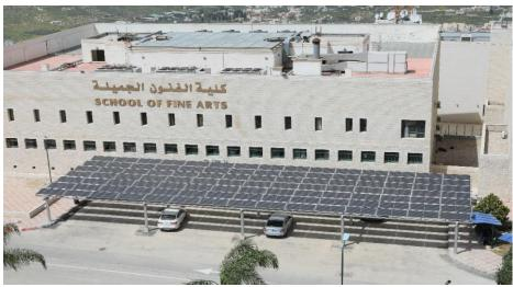
Fig.2 PV carport-new Campus PV system
