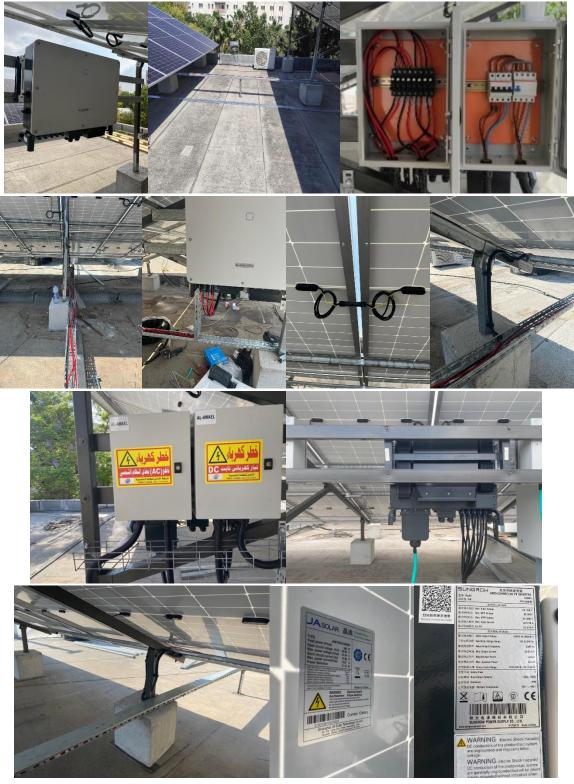
6- Then the DC/AC earthing was connected and lightning Pulsar, Earth resistance measurement 2.8 ohm
