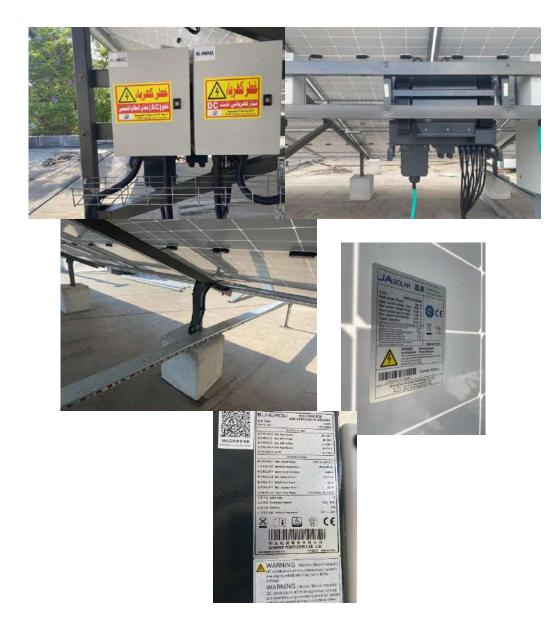
26-Then the DC/AC earthing was connected and lightning Pulsar, Earth resistance measurement 2.8 ohm
