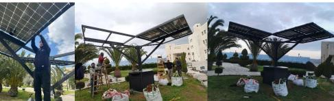
5- Install inverter/charger and connect all components and all the cables were installed in tranches and trunks for aesthetic image of the project and facilitate the maintenance work in future
