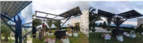
17-Install inverter/charger and connect all components and all the cables were installed in tranches and trunks for aesthetic image of the project and facilitate the maintenance work in future
