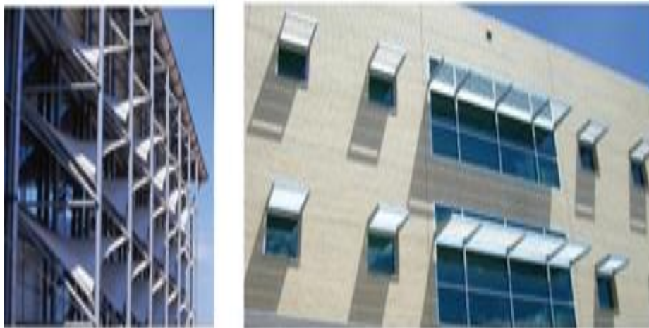
Figure 35: Proposed solutions for external shading according to a local study
