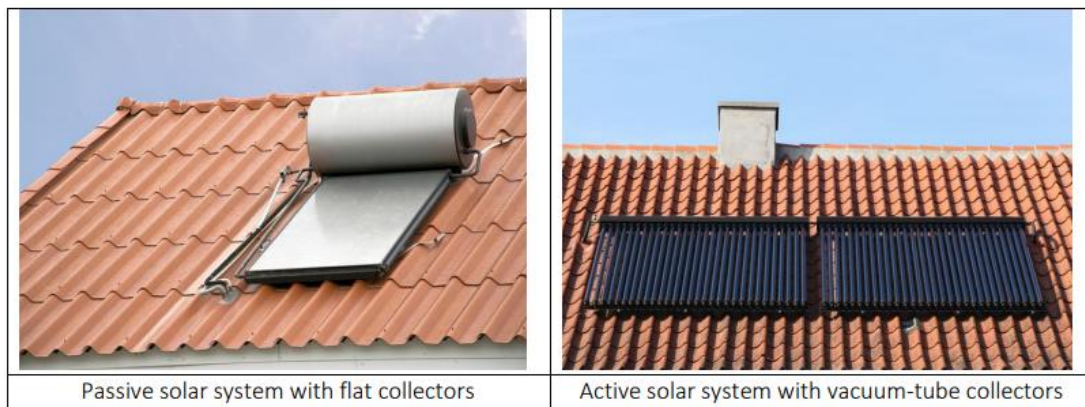
Figure 8: Examples of solar heating systems
