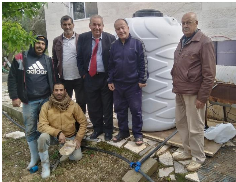
Figura 46. Installing irrigation system for UA
