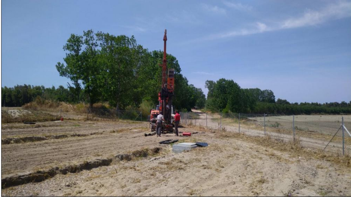
Figure 49. Realization of the core drilling S1
