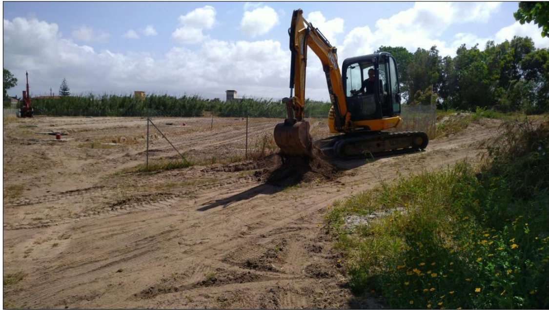
Figure 46. Realization of the geognostic test-pit P1
