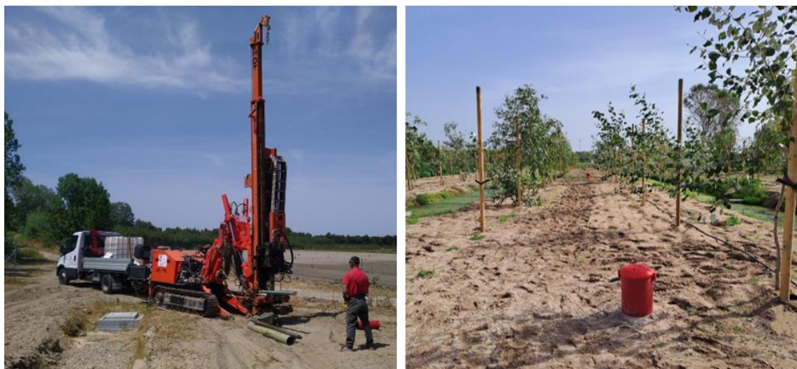
Figure 37. Drilling and final setup of the piezometers
