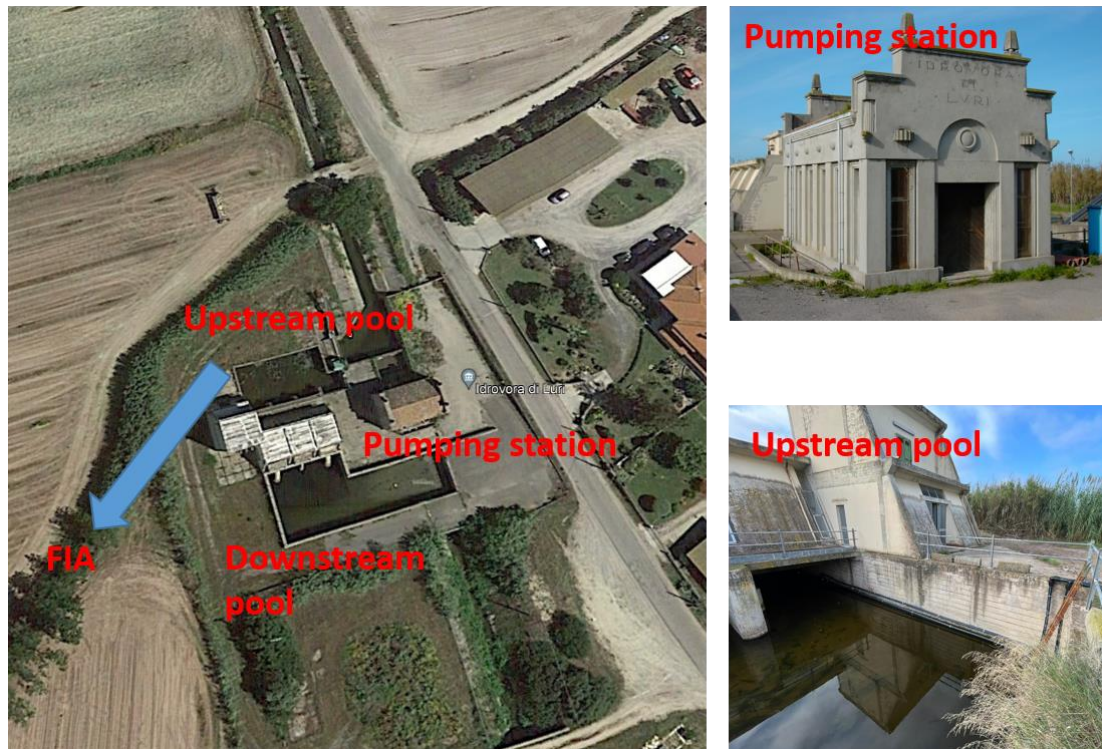
Figure 14. Overview of the dewatering pumping station of Luri, in Arborea
