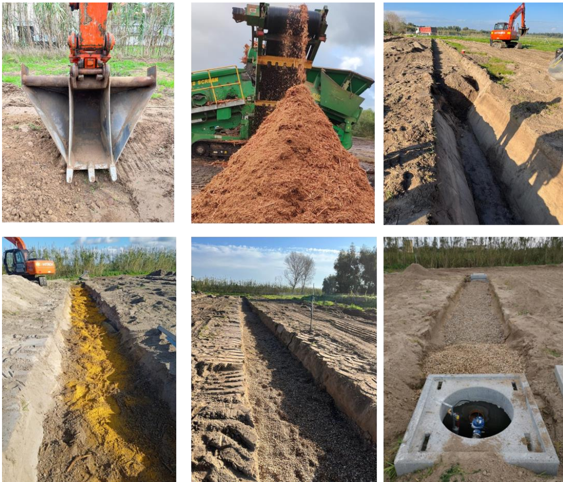
Figure 31. Phases of construction of the PTS in the excavated trenches
