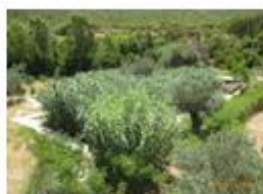
Jougar wastewater treatment facility
