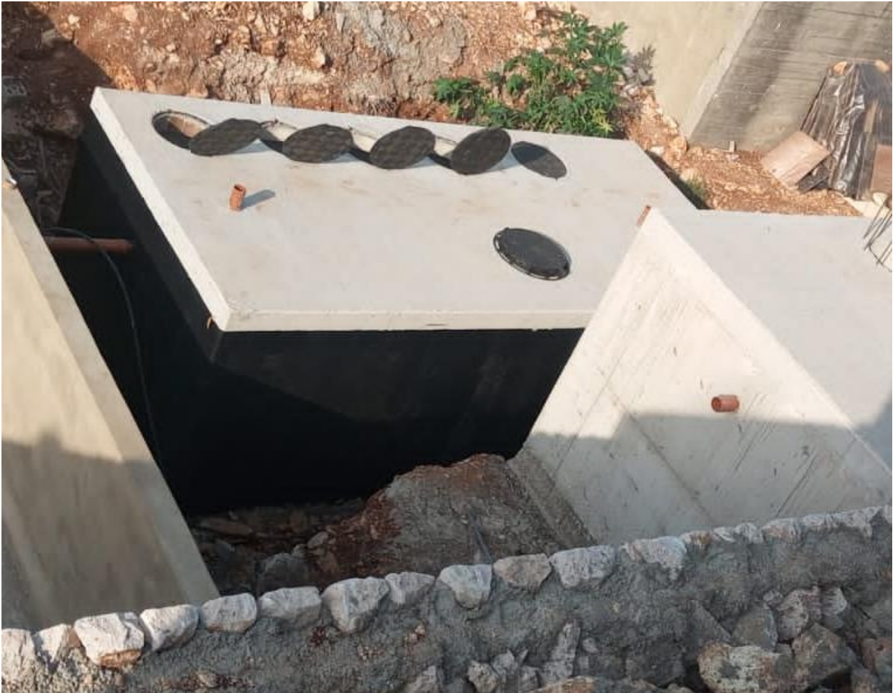
Figure 51. Anaerobic Baffled Reactor.
