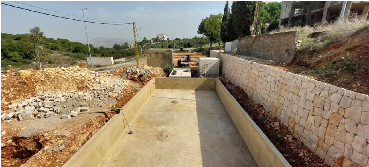
Figure 52. Constructed wetland.
