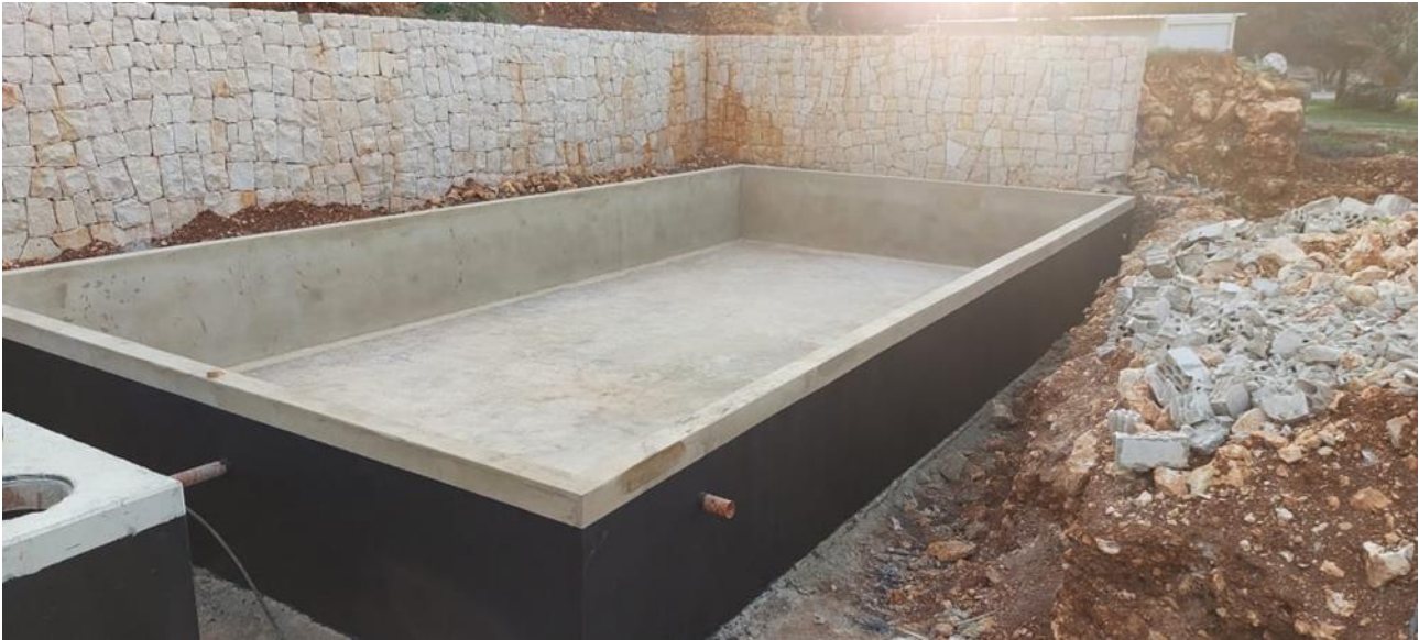
Figure 45. A detail of constructed wetland.
