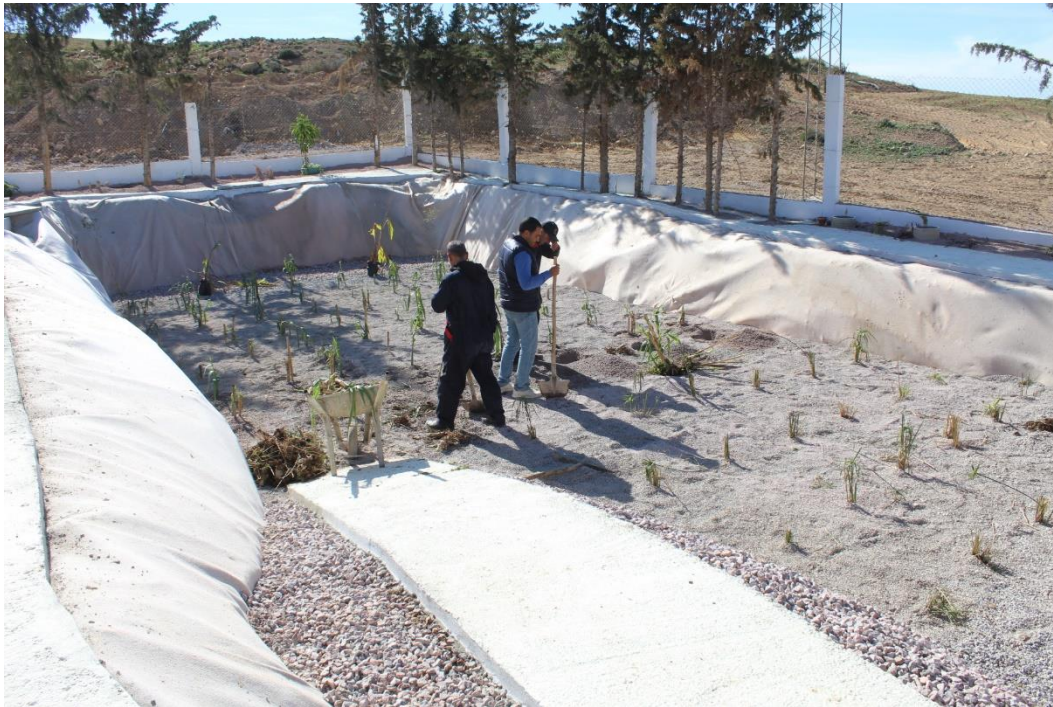
Figure 61. Sowing of plants in the horizontal wetland
