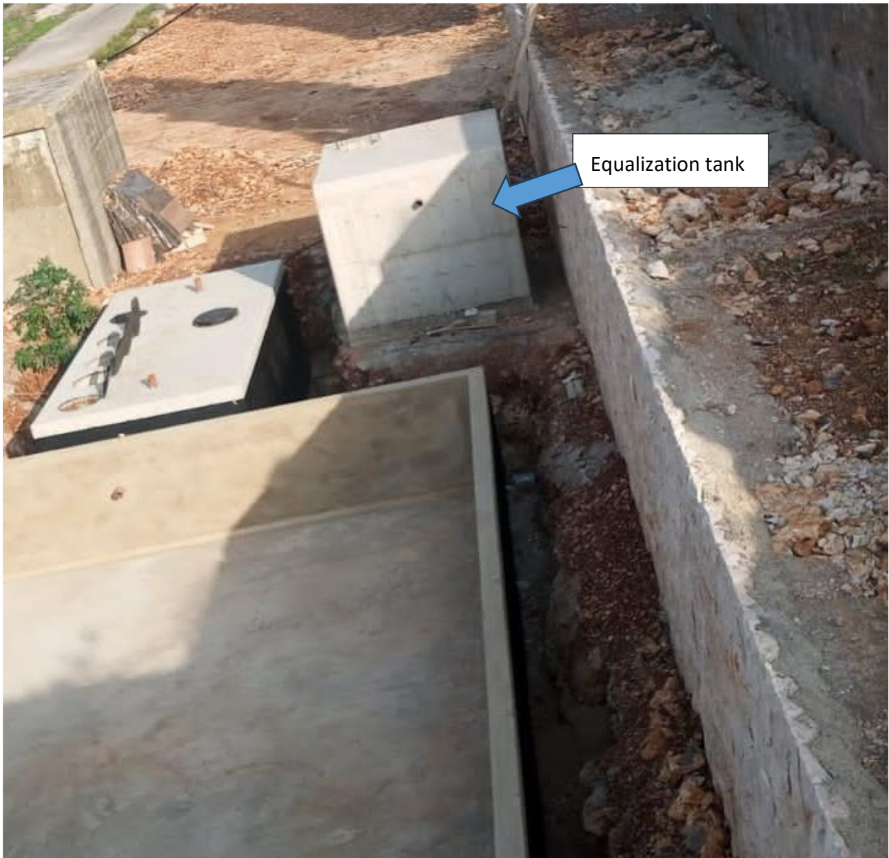
Figure 44. Equalization tank.
