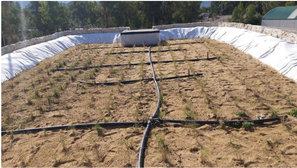
Figure 17. The horizontal wetland.
