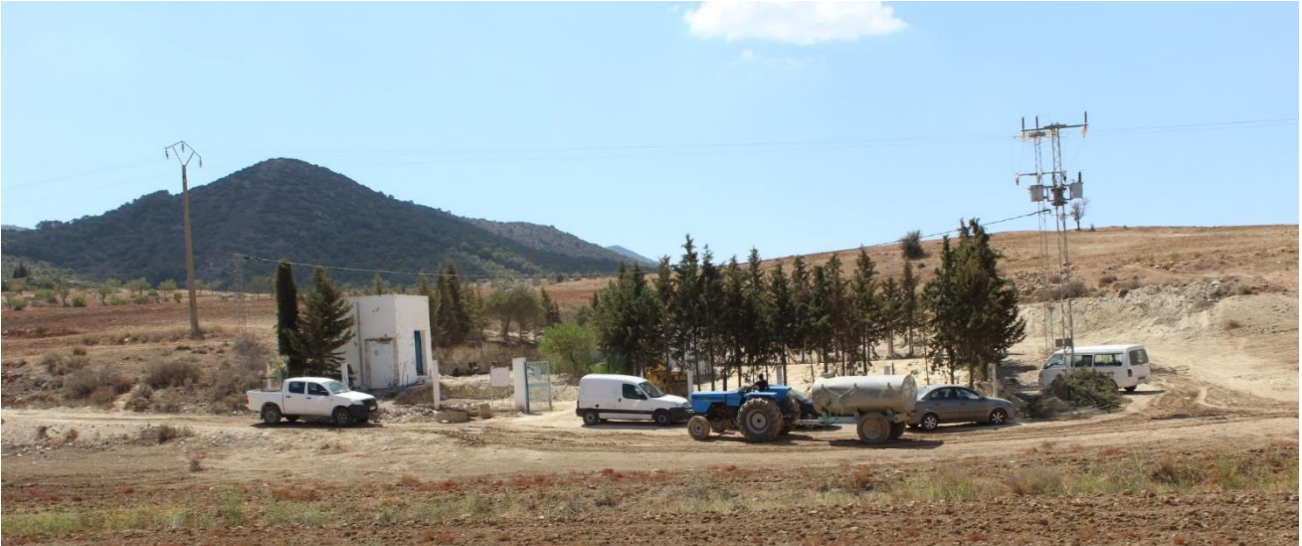
Figure 55. Location of demo site plant
