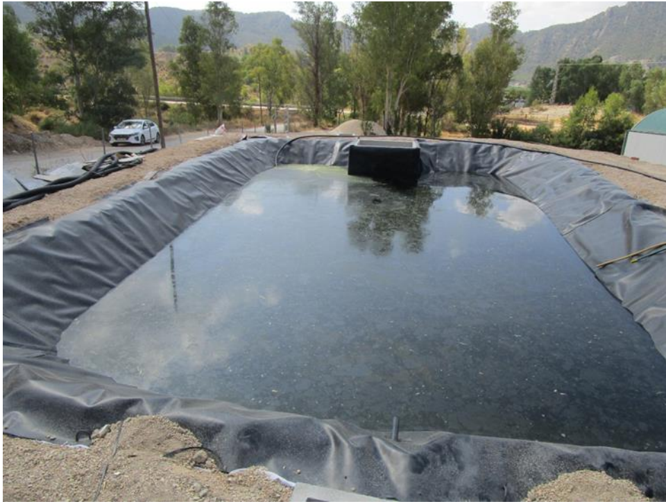
Figure 11. Test to check the impermeability of the wetland.
