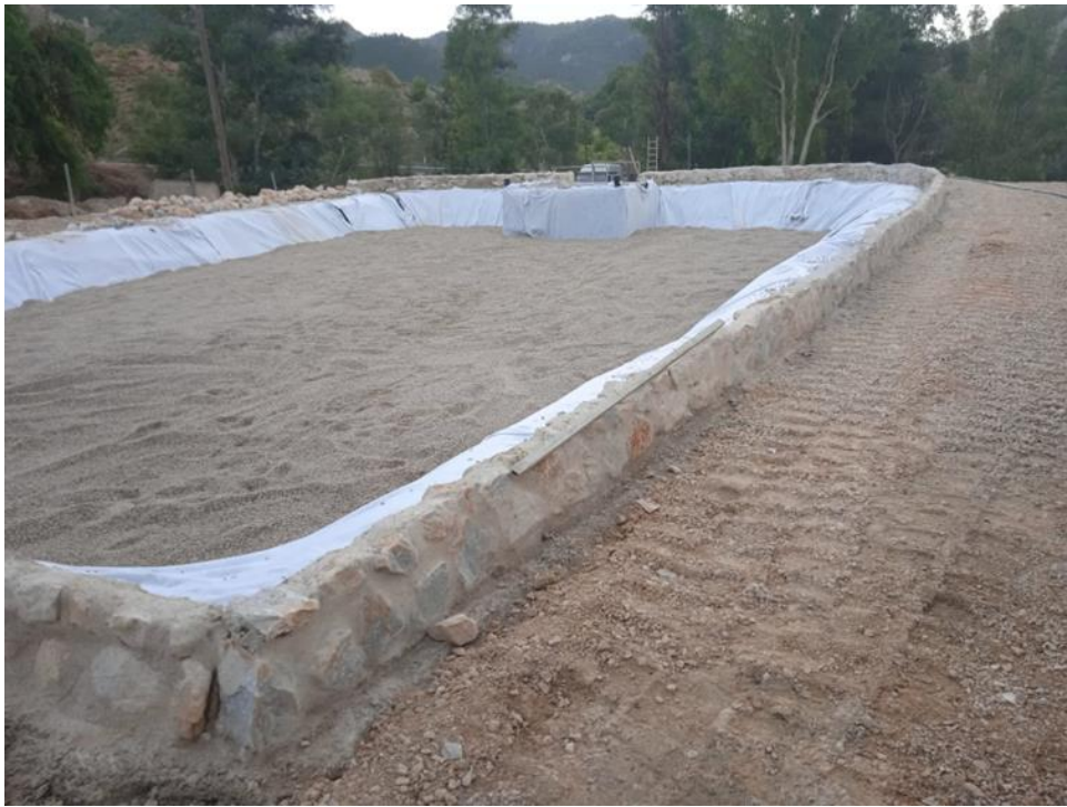
Figure 15. The vertical wetland once the filling process has finished.
