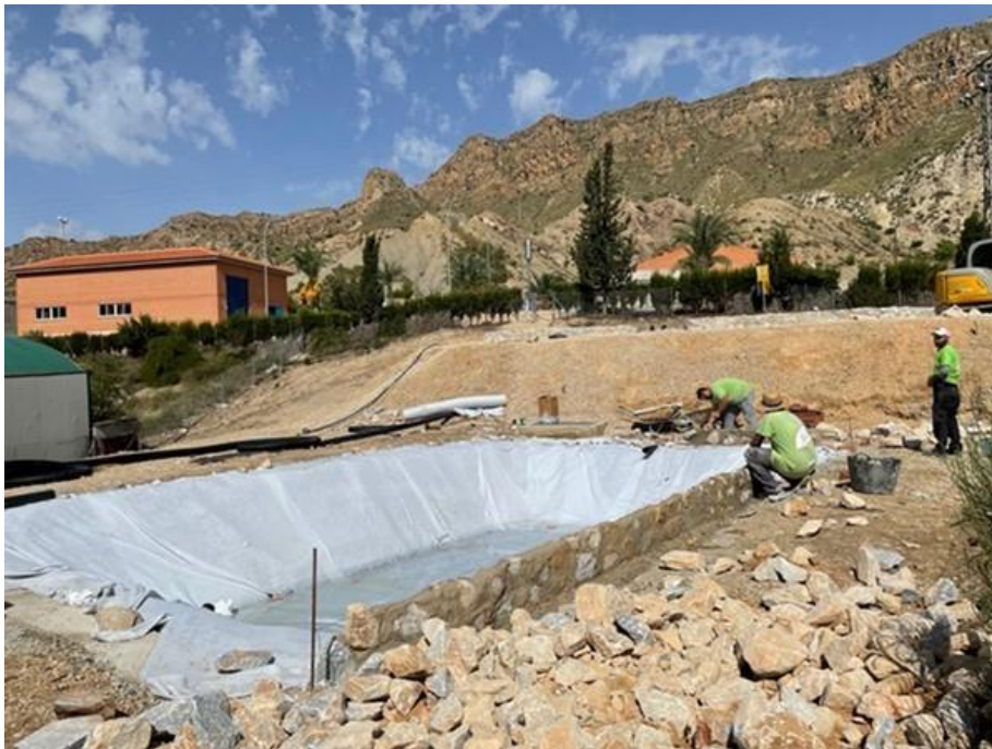
Figure 11. Test to check the impermeability of the wetland.
