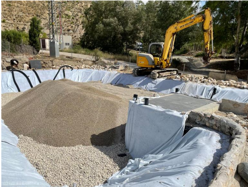
Figure 13. A detail of the granular material filling process in the vertical wetland.
