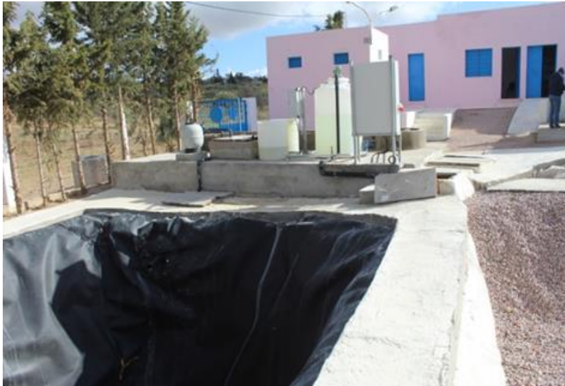
Figure 65. Storage basin, for the treated water
