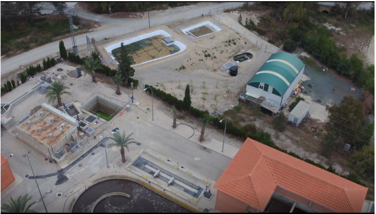
Figure 2. The real demo-site plant.
