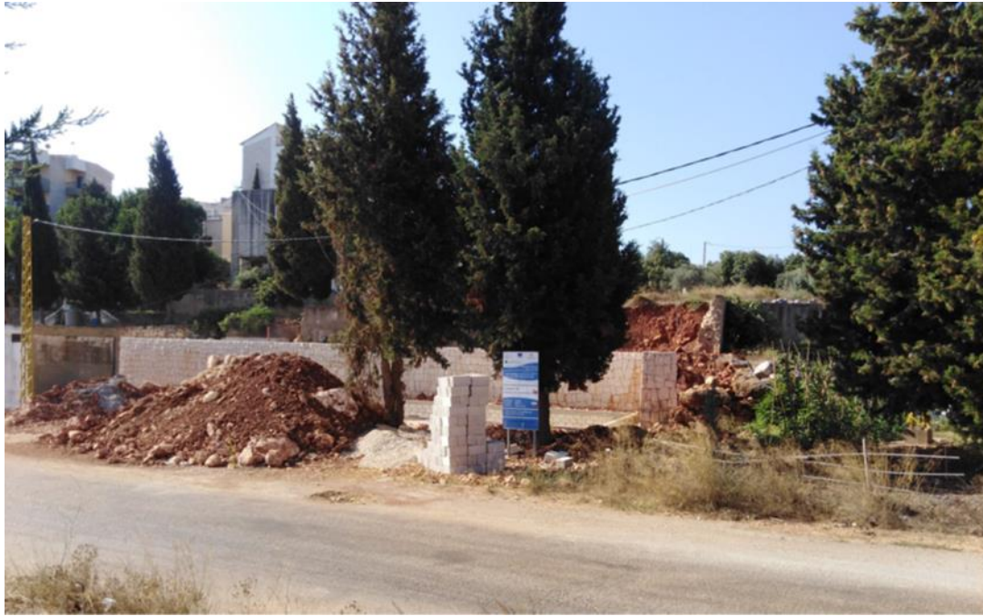
Figure 42. First steps of the construction.
