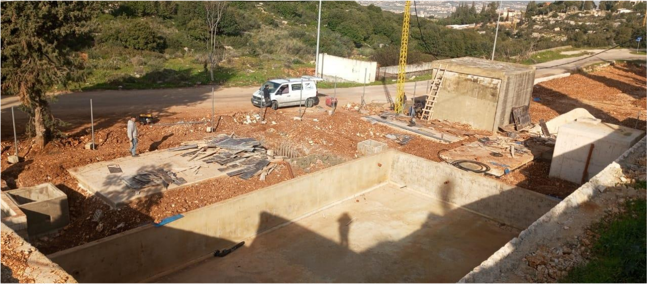
Figure 49. Land filling completion.
