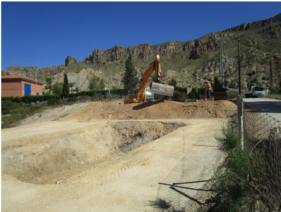
Figure 8. A detail of the excavation of vertical wetland.
