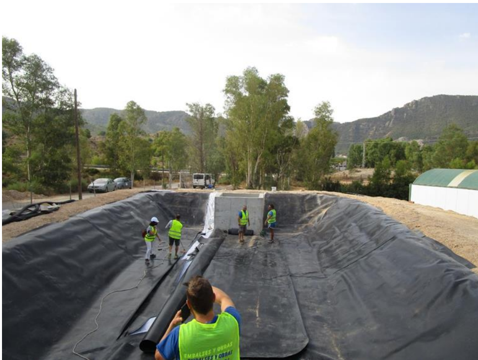
Figure 10. Installation of geotextile.
