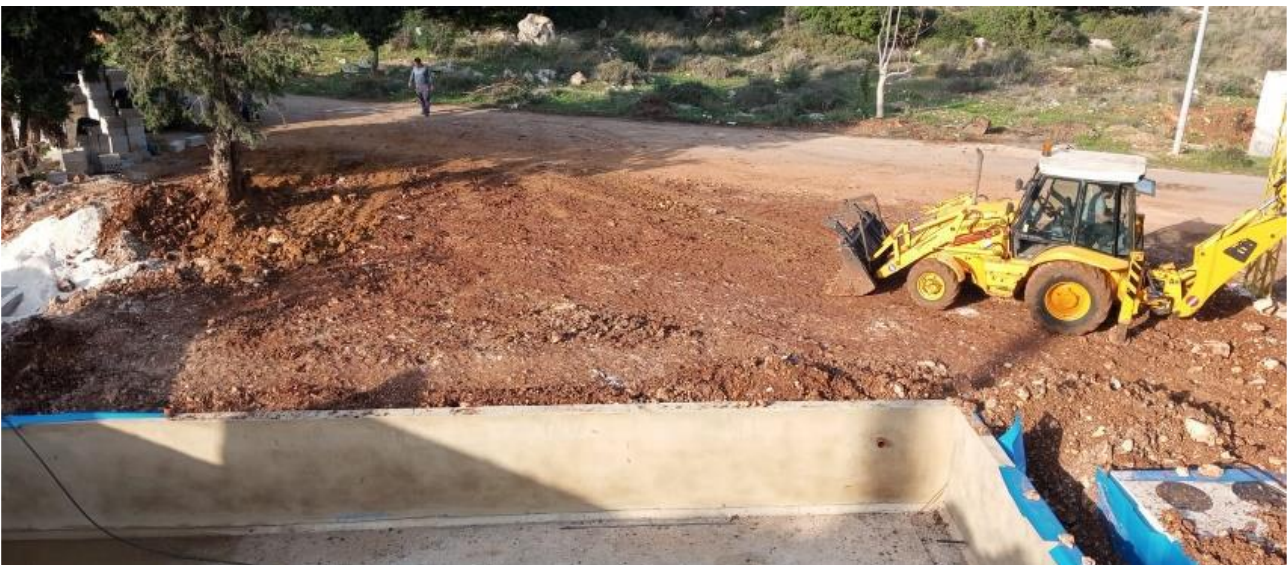
Figure 48. Some detail of the construction.
