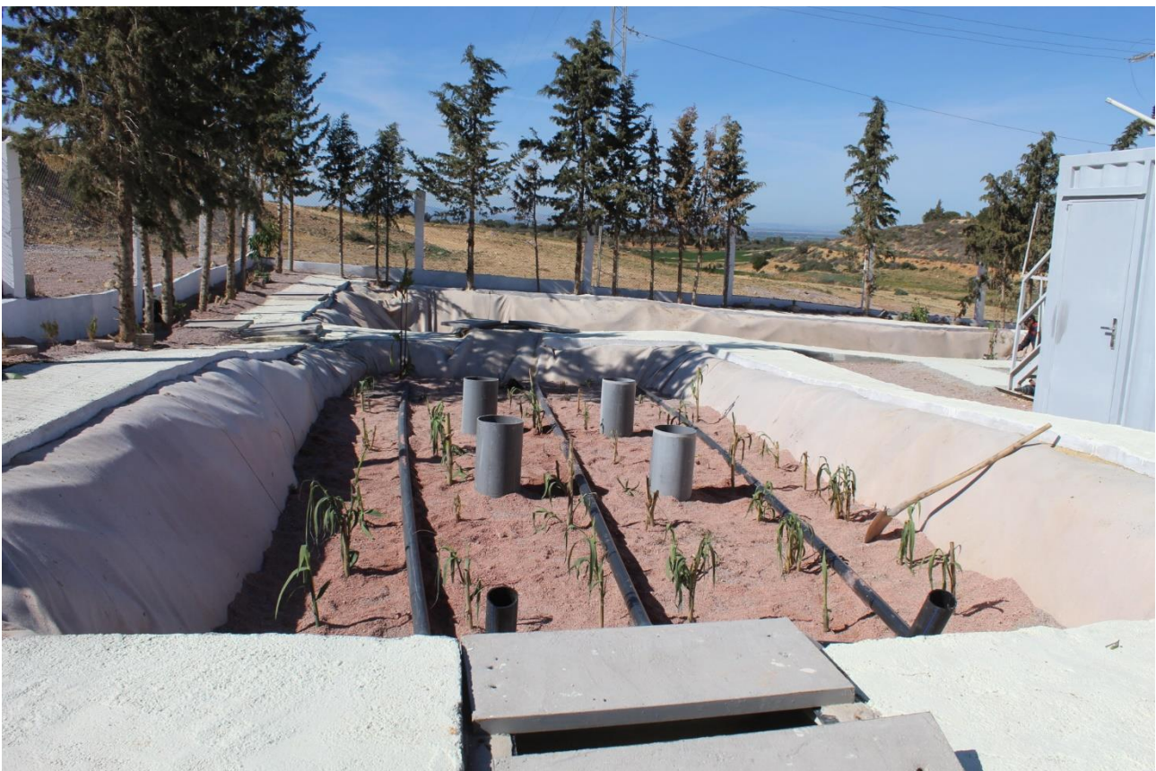
Figure 62. Vertical and horizontal wetlands
