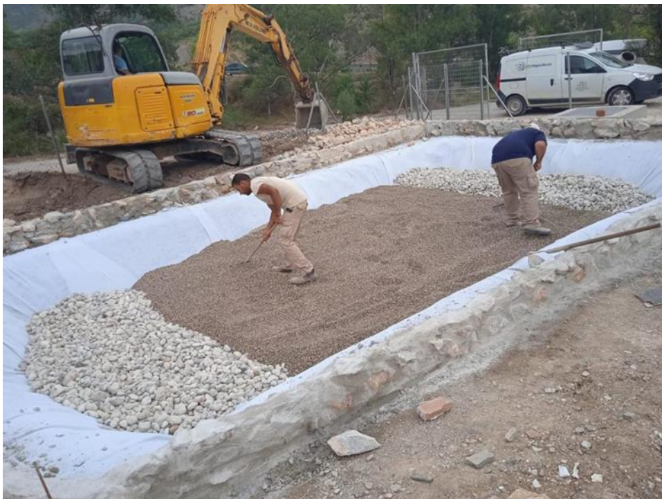
Figure 14. A detail of the granular material filling process in the horizontal wetland.
