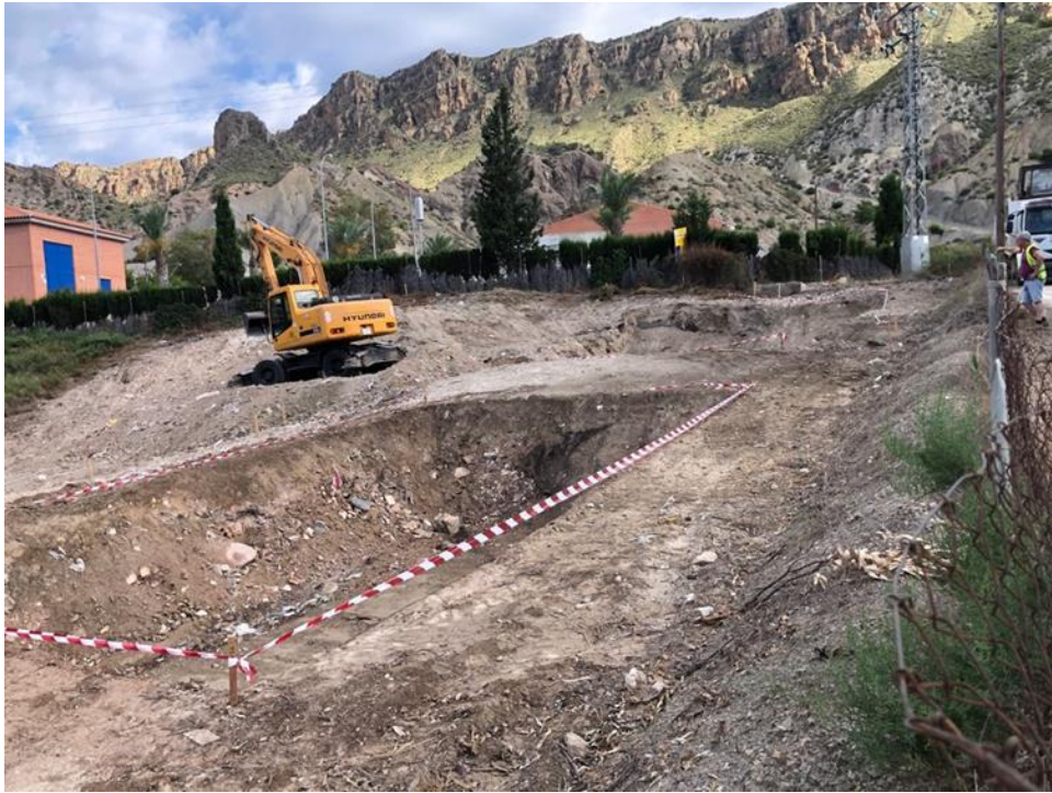
Figure 7. The excavation of vertical wetland.
