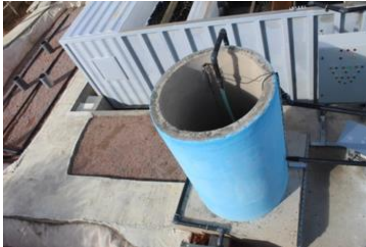
Figure 59. Settlement tank.
