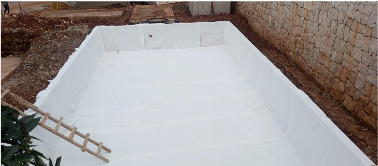
Figure 50. Installation of the wetland membrane.
