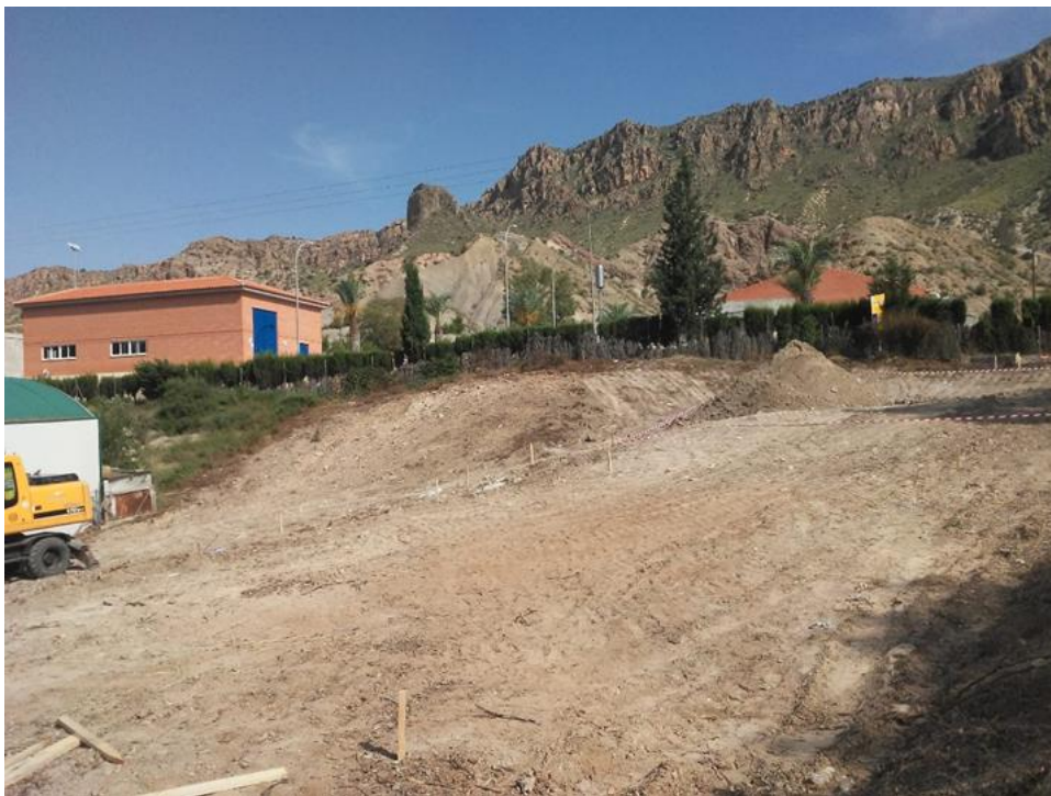
Figure 6. The start of excavation.
