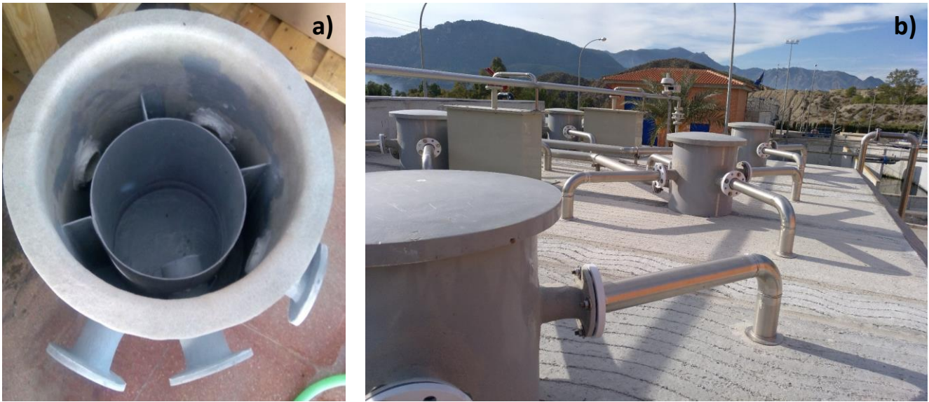
Photo 1 a) Inlet of a single distribution system unit, b) view of the integrated distribution system.
