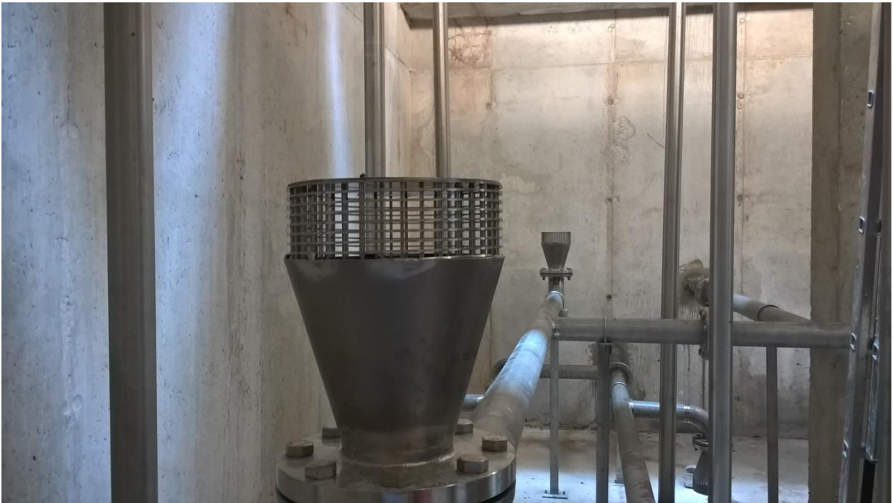
Photo 4 Sludge withdrawal system.
