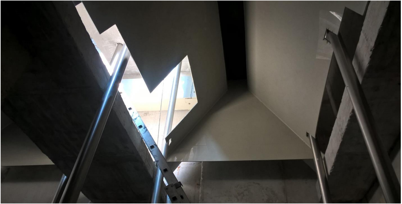
Photo 3 Three phases separator.
