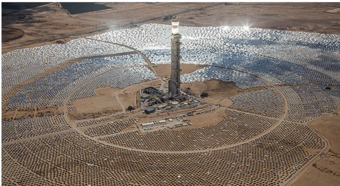
Figure 22: Ashlim Solar Power Plant
