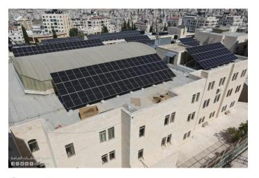
In the framework of Med-EcoSuRe project, photovoltaic solar power plants were installed on the roof top of different buildings at An-Najah National University, Palestine with a total capacity of 165 kW.
